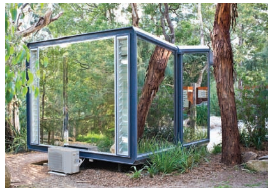
'Zoo Booth' displays an innovative use of mirror finished grade 304 stainless steel and (bottom), from inside a Pop-up home office space assembled in a suburban back yard.
